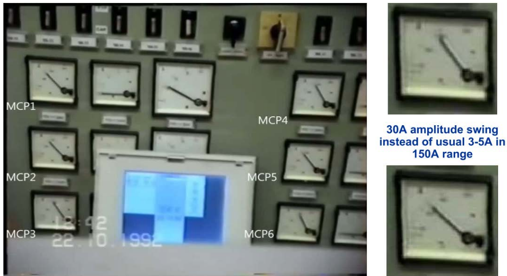
Figure 51. NPP Dukovany Unit #4 MCP supply current fluctuations
