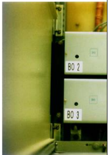
Detail of optical isolation units
